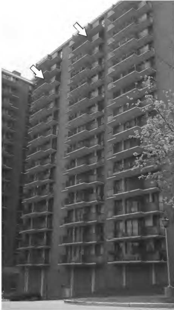
Fig. 1. Arrows mark the location of hummingbird feeders on the balconies of a high-rise apartment building in College Park, Maryland. The highest feeder was 43 m above ground level.
